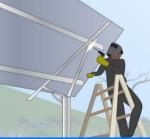
**WELD** the steel bolt/screw to the steel support frame (but taking into account that it will be difficult to remove he modules in case of replacement need).
